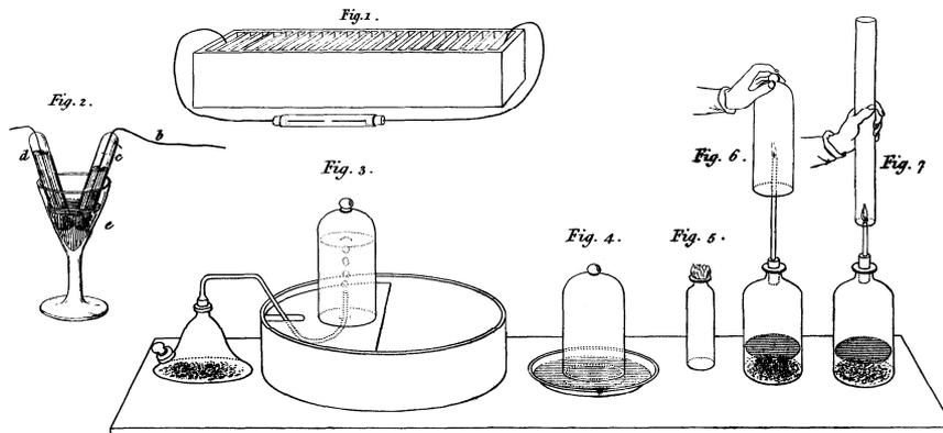
Figure 3: Apparatus for decomposing water and studying hydrogen (from Marcet 1828, plate XI).
