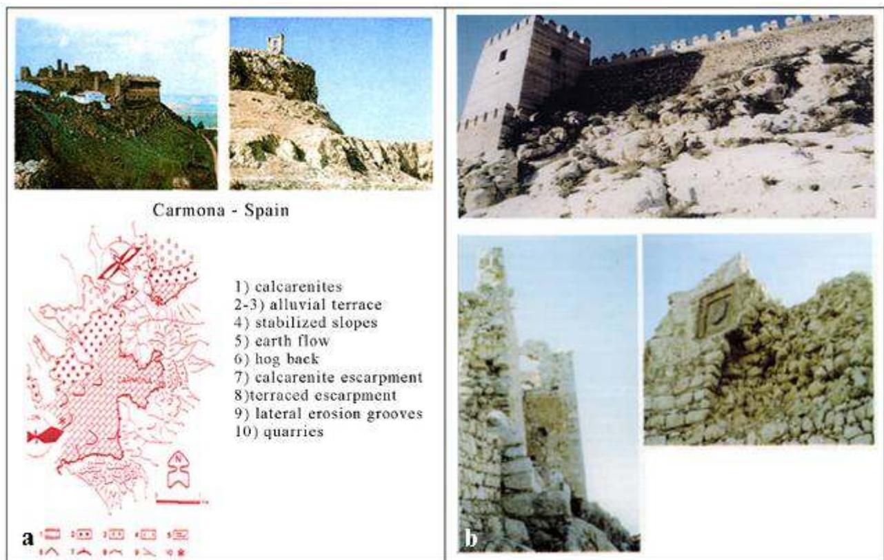
**Figure 8:** Neotectonics and slope movements: a) failures affecting the Castle and the Tower of Carmona (Spain) due to the dynamic of the slopes; b) effects of seismic activity on walls weakened by marine spray action on mortars (Castle of Kalki, Greece) or intensified by the steepness of the slope and the elastic behaviour of fissured rock (Alcazaba the Almeria, Spain).
