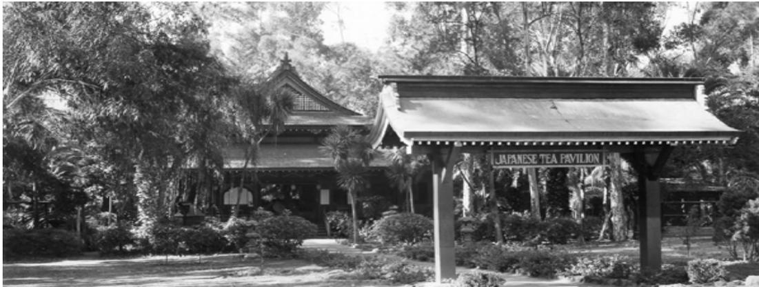
Though the building in Balboa Park appeared to have two roofs, it was a one-story building with an intermediate or pent roof, shielding an open verandah. Both roofs were covered by wood shingles rather than tiles. The main hip and gable (irimoya) roof with its curving eaves, was as striking as a woman's colossal hat. The entrance was on the lateral side of the building, not, as is common in Japanese temples, on the narrow or gable side.
